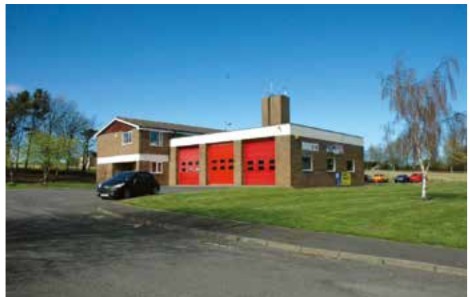
Berwick Fire Station as existing
