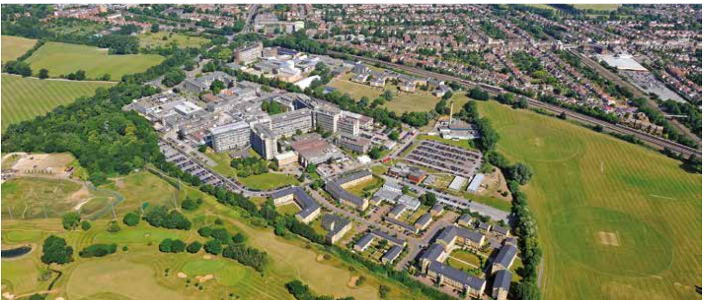
Northwick Park, aerial view
